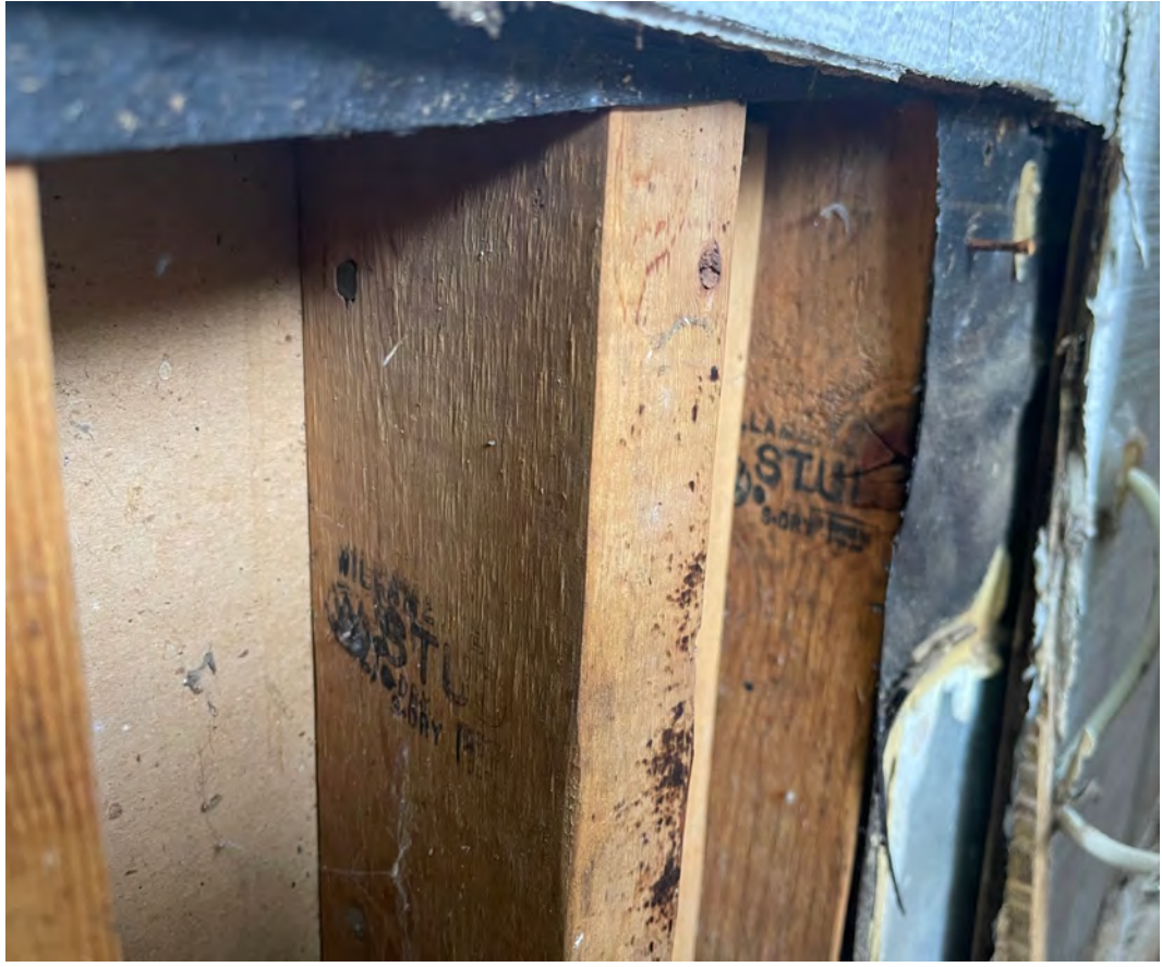
MODERN STUDS AS INDICATED BY LUMBER STAMPS AND NAILS
