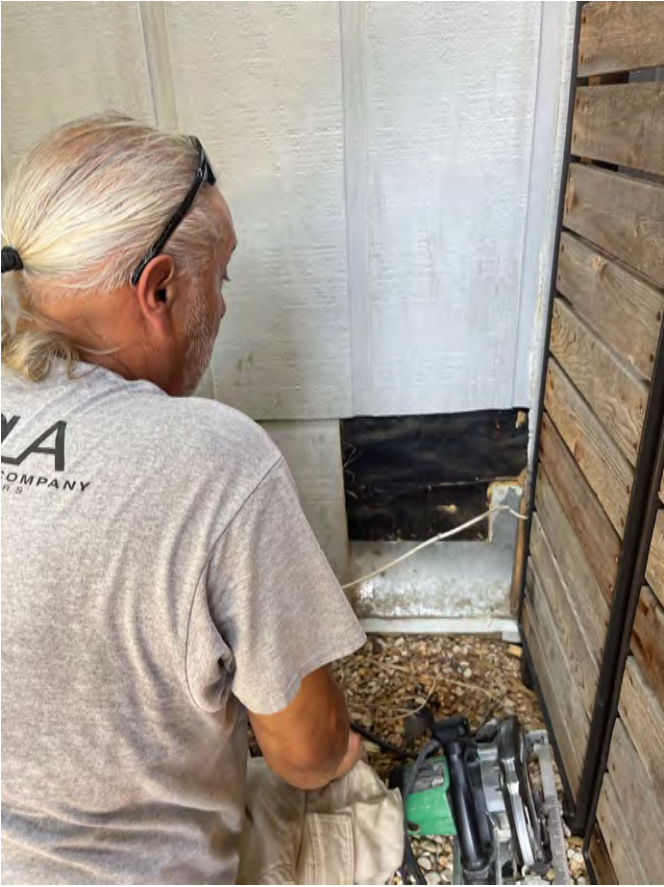
BLACK FELT PAPER BEHIND T111 SIDING
