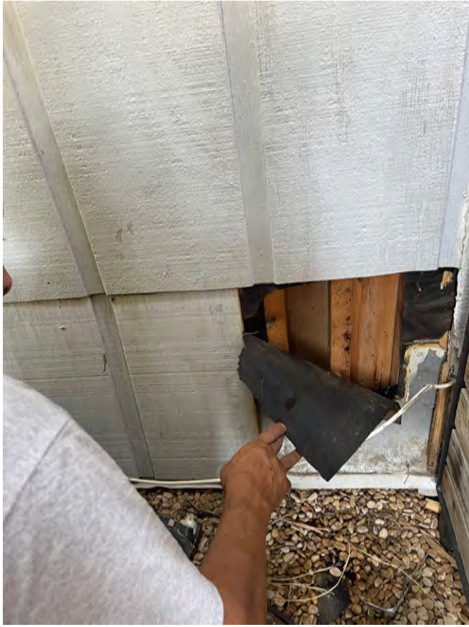
WOOD FRAMING BEHIND FELT
